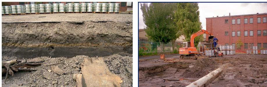
Figure 2: Removal of material from car park at Fisherman's Bend (Victoria) in 1990. Approximately 10,000 drums each 200 L were filled with soil and rubble, then temporarily stored at ANSTO until being transferred to Woomera in 1994/5.
